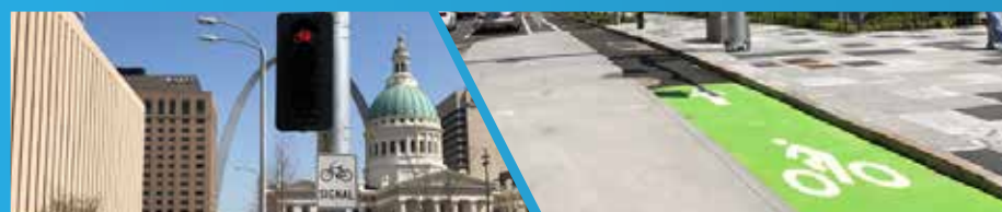
Improvements to the Chestnut Street bikeway included curb-protected intersections and segments, as well as one of the region's first bicycle signals.
